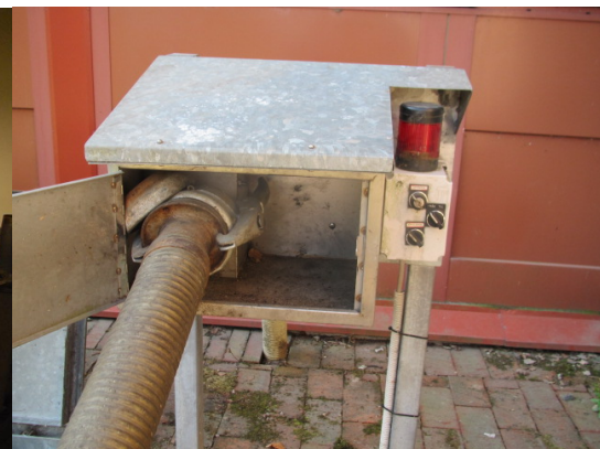
Terminal for extraction truck
